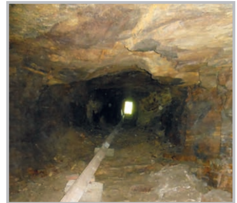
Blick in den Tunnel 2015“
